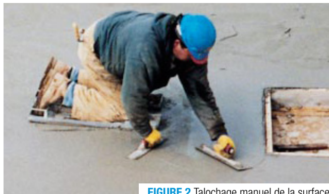
FIGURE 2 Talochage manuel de la surface
