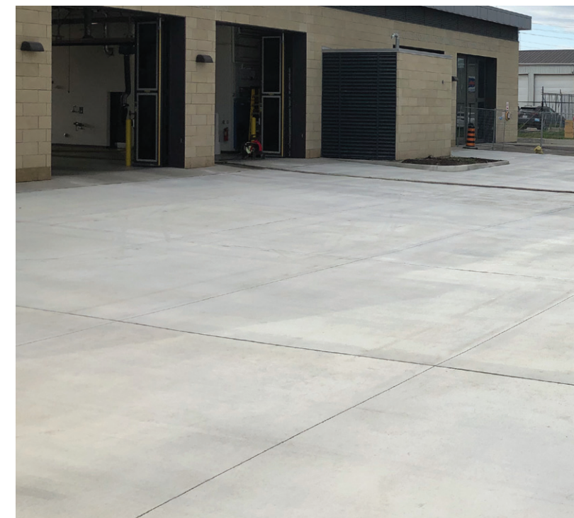
City of Vaughan Fire Station 7-3 and EMS Station 31 Parking Lot in 2019
